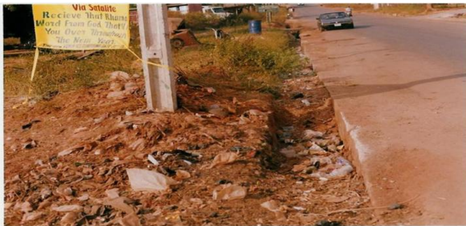
Plate 5: Drainage Blocked by Solid Waste
