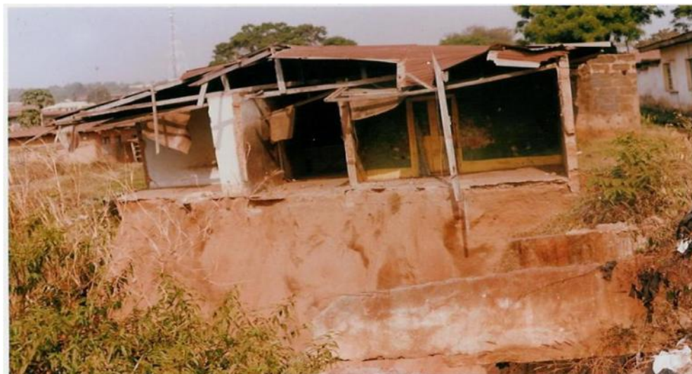
Plate 3: Residential Land Use Totally Destroyed By Soil Erosion At Akpeke Quarters
